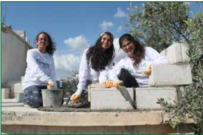
ISC-Amman student volunteers building a shelter for a family in need
